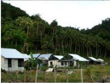
JRS house rebuilding project for the Meulingge village in Pulo Aceh
